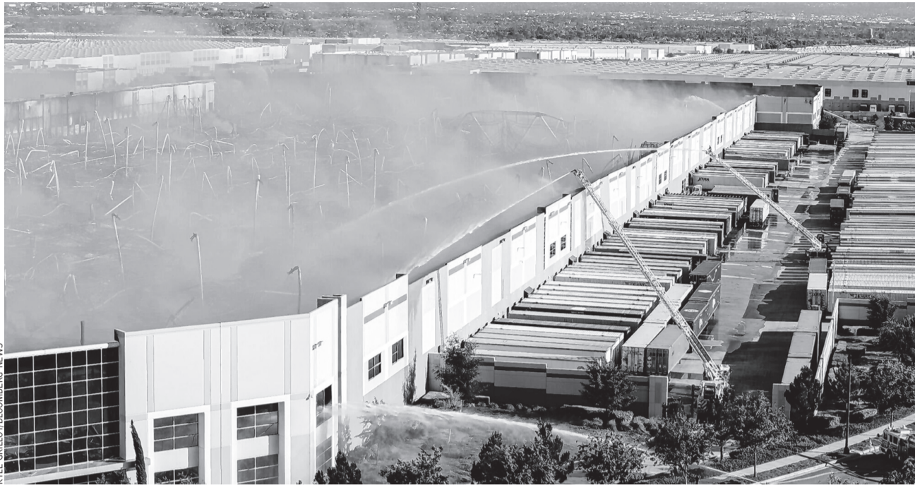
A fire set this month at an Ontario, Calif., warehouse storing Kimberly-Clark products caused about $500 million in damage.
